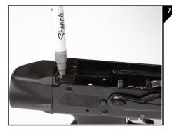
Next, use a paint pen to mark a circle onto the mount by placing the pen through the exisitng hole in the receiver as seen in Figure 2. Make sure the mount is held tight and flush to the receiver when making your mark.
